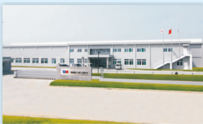
合肥 第2工厂 (软管单体、金属接头) Hefei No.2 Plant ( hose & coupling production )
